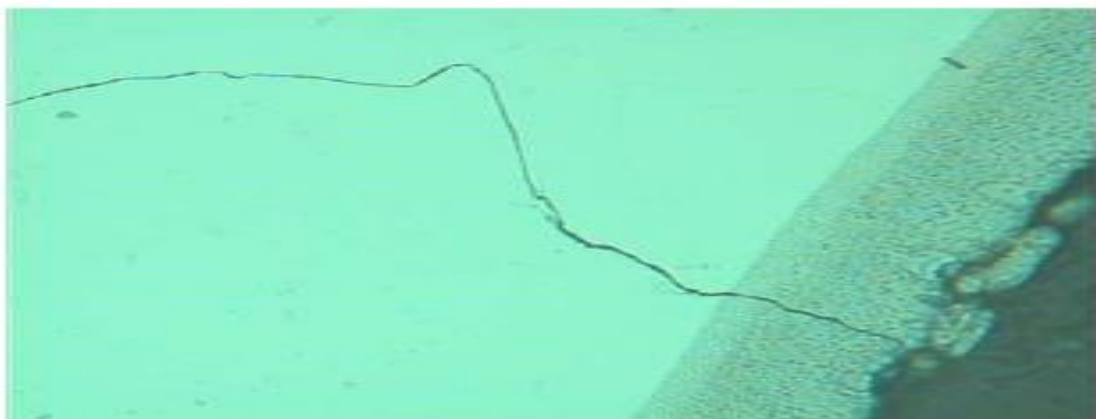
Figure 1.11 – Protective-coating cracking; the crack keeps propagating into the blade's native material
