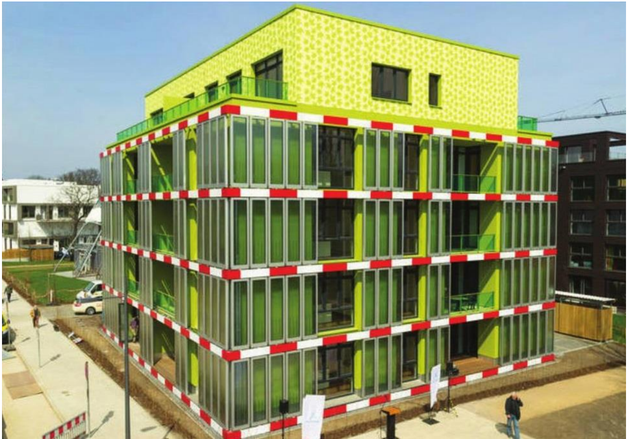
Figure 2.3. The first experimental house BIQ house, which generates energy using microalgae panels located on its facade (Hamburg, Germany)
