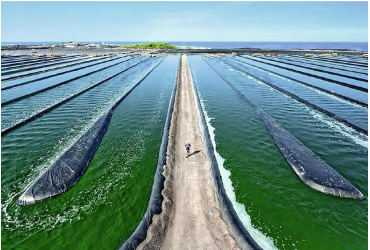
Figure 2.6 Open algae biomass cultivation system
