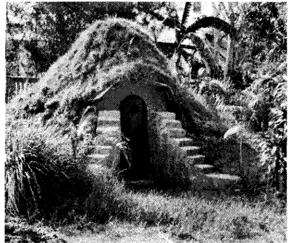
Fig. 5. Example of earth-bag construction
