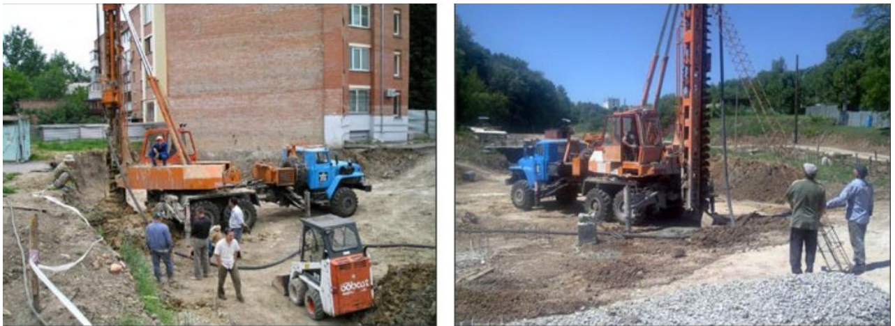
Figure 4.2 - Drilling wells for bored injection piles
