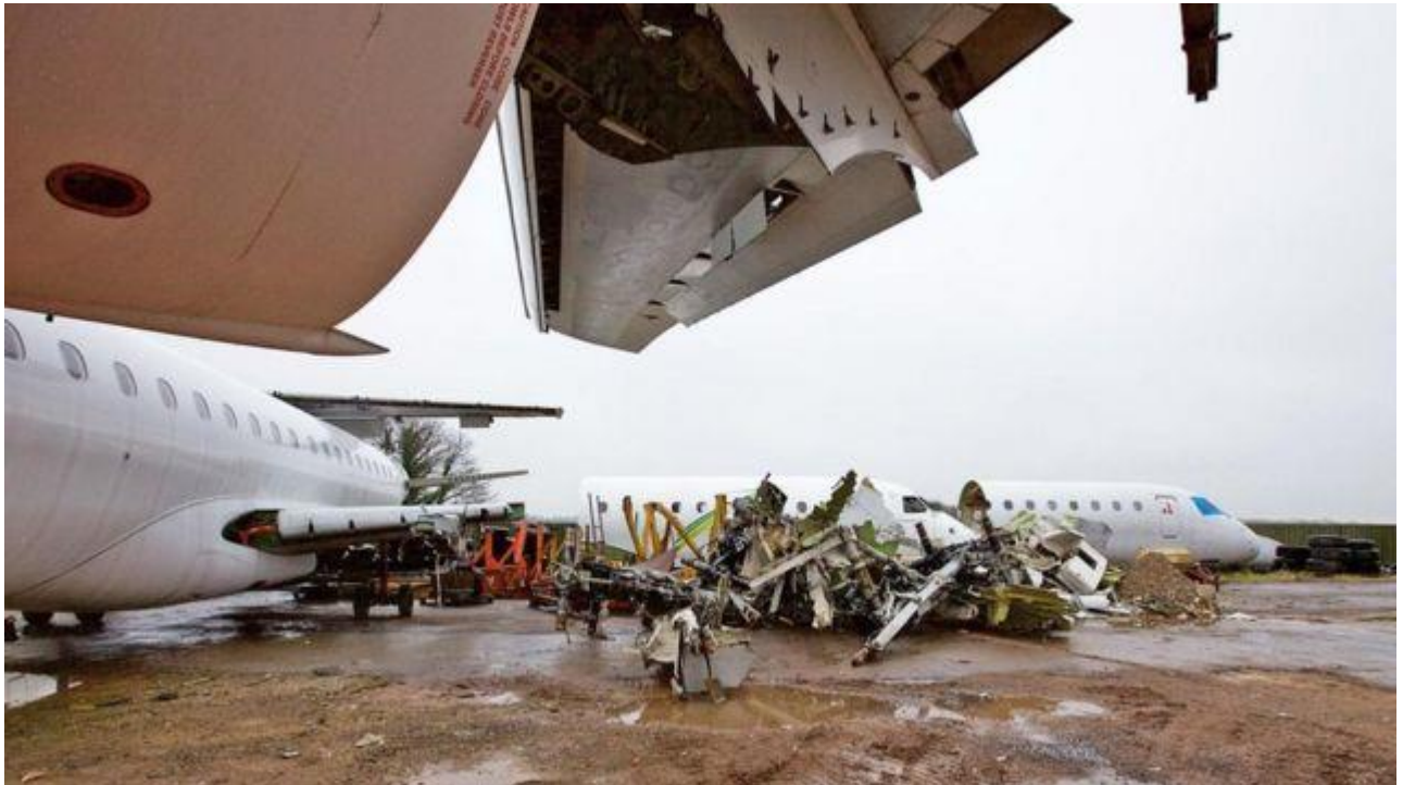
Fig.3.5 - Commercial aircraft dismantling site
