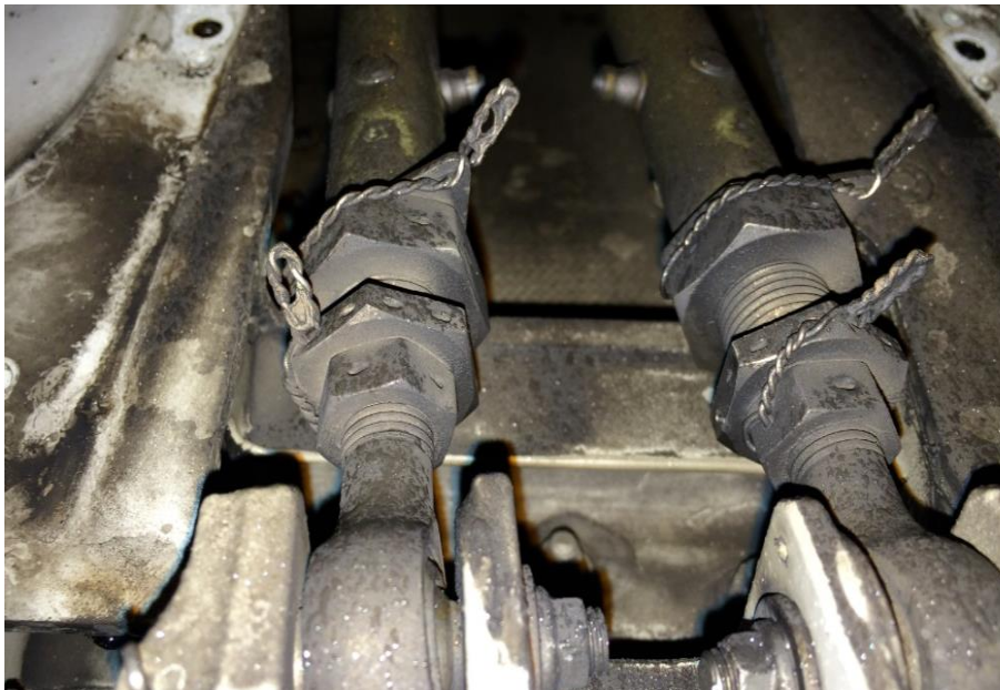
Fig. 1.10 - Corrosion was found on the inner flap control link
