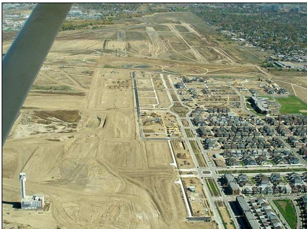
Fig.3. The process of dismantling of the airport, 2003 [6]
