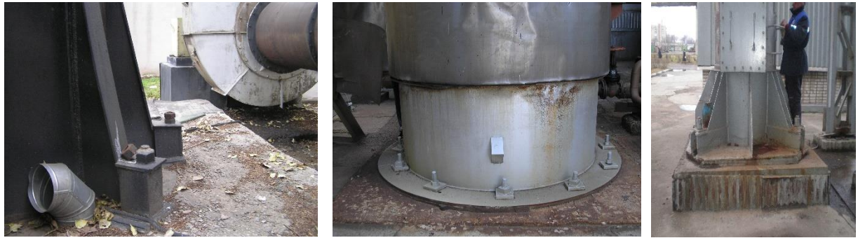
Fig. 1.2 Support units of metal chimneys:
