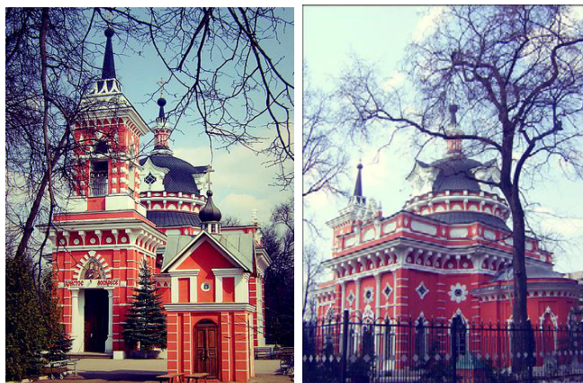
Figure 24, 25. The Church of the Saviour. Ivanteyvka. E.O. Batashev manor. 1808 Architect A.N. Bakarev (?). View from the southwest (left). View from the southeast.
