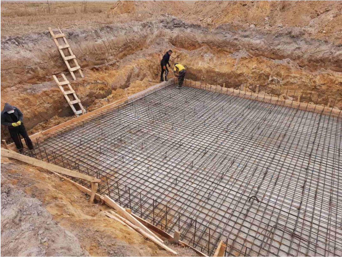
Fig.2. The beginning of the first phase of construction
