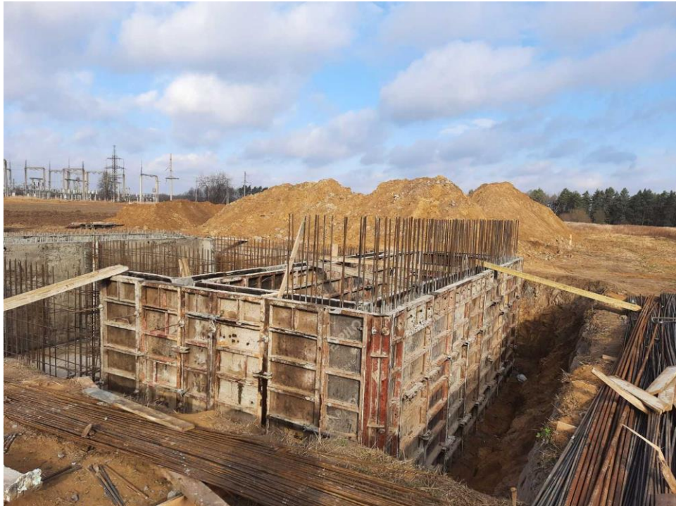
Fig.5. Pouring concrete structures
