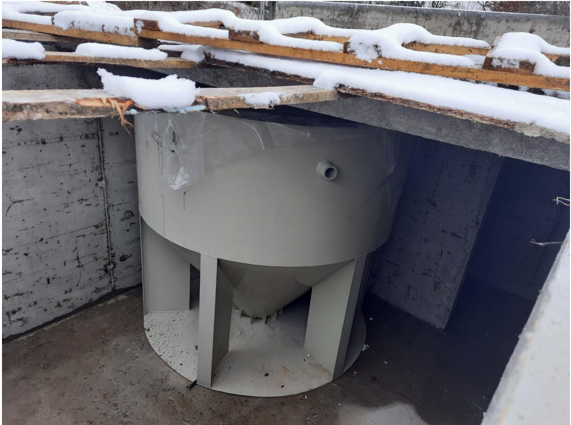
Fig.7. Installation of the equipment of two clarifiers without mechanisms
