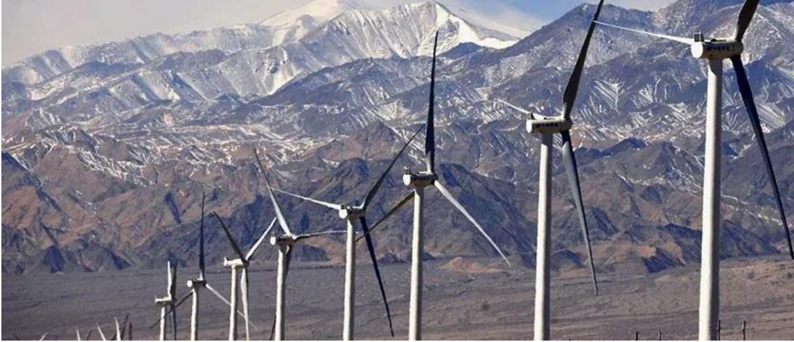
Fig. 5.3. Wind power generation device.
