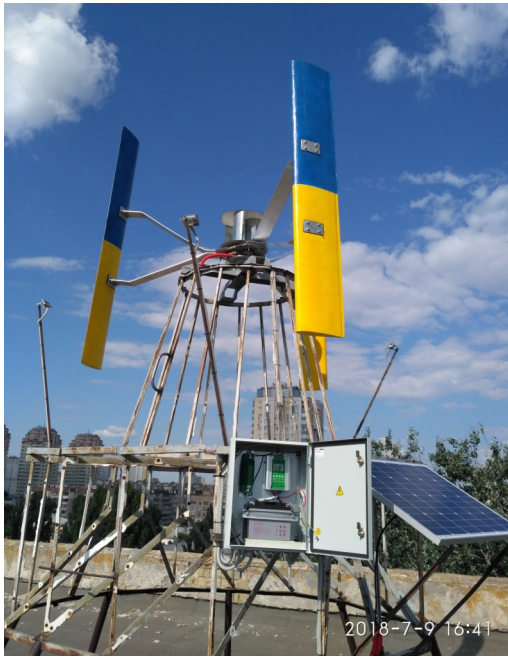
Fig. 3. Hybrid power plant
