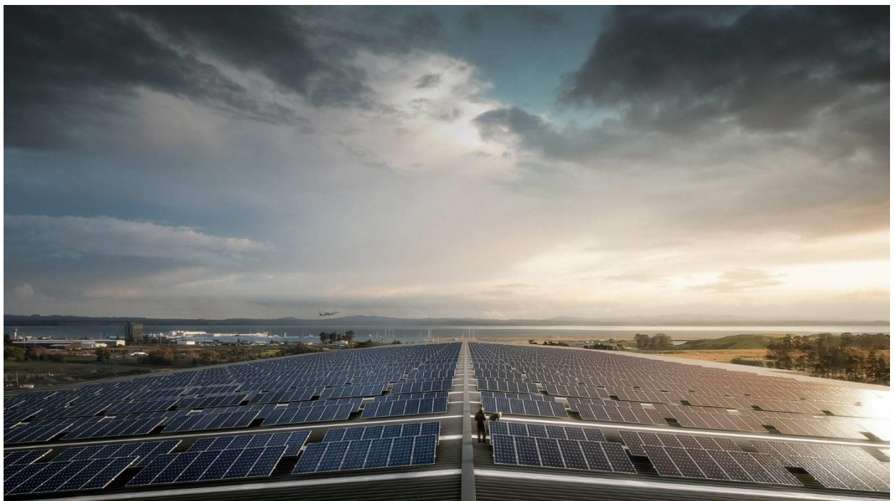
Fig.3.6. Location of solar panels on the roof
